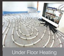
Radiant Panel Heating
